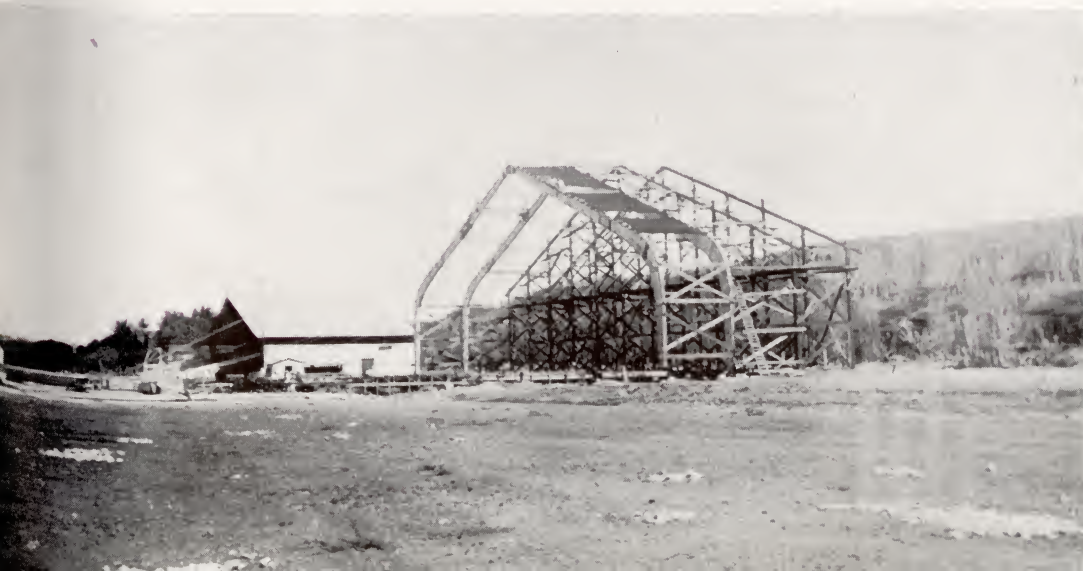
Hangar No. 2 is gradually proceeding, August 1935
